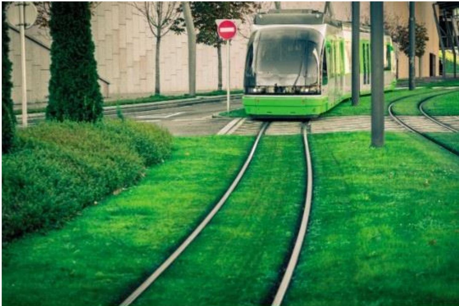
**Planting vegetation along light rail tracks is possible, help filter rainfall and reduce flooding, runoff would contain less pollutants than if it had fallen on hard surfaces such as concrete**
